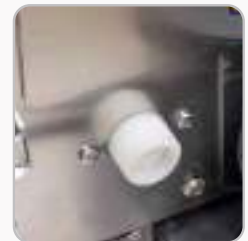
Water mains connection
