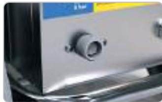
Water mains connection
